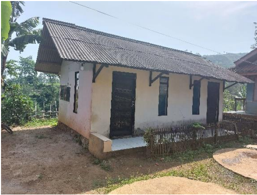
Figure 20. Typical housing in Pacet
